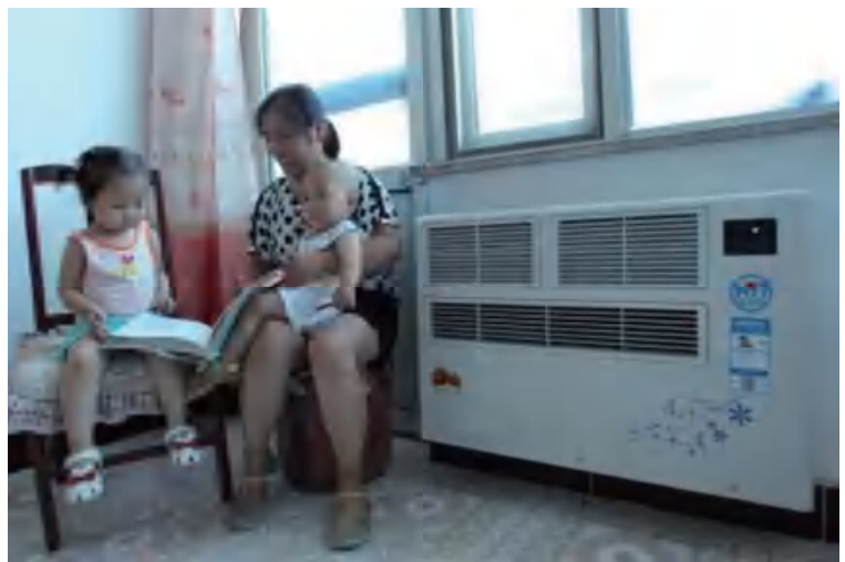
Indoor unit of geothermal energy heater in a villager's home
